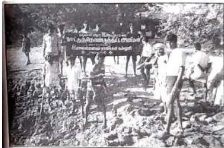
NSS Volunteers at Work - Repairing a Bridge
